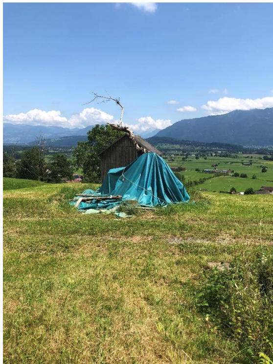
Blick abwärts, km 0.510
